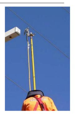
Using the same method, cock each of the three clamps on the phase/shorting lead set and fit into the three sockets on the platform. Apply this set with the same smooth downward motion as before, until each clamp separates from the platform. When fitting the clamp to an outer phase, make sure the removal eye at the top of the clamp is towards the center phase i.e. the open mouth of the clamp is facing outwards.
