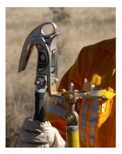
Using the operating rod, position the earth lead clamp above the phase conductor to which the earth lead is to be attached preferably the centre phase, and with a smooth downward motion, pull the clamp onto the conductor until it triggers and snaps on to the conductor, continuing the downward motion until the clamp has separated from the platform.
